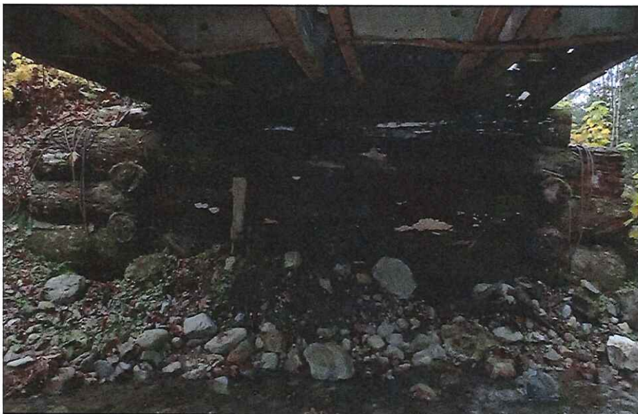
CK2253 Left Abutment
